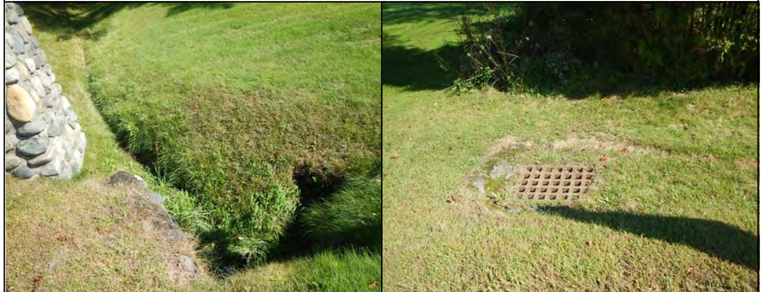
Photo 1. Narrow ditch that needs to be expanded. Photo 2. Erosion around catch basin.
