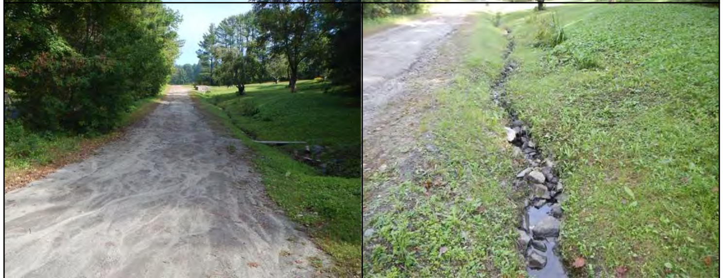
Photo 1. Easy Street and roadside ditch to the right. Photo 2. Ditch in need of repair.
